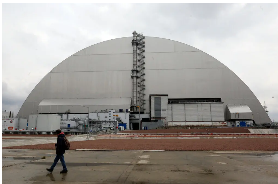
The safe confinement covering over the No. 4 reactor in 2021. Efrem Lukatsky/Associated Press
